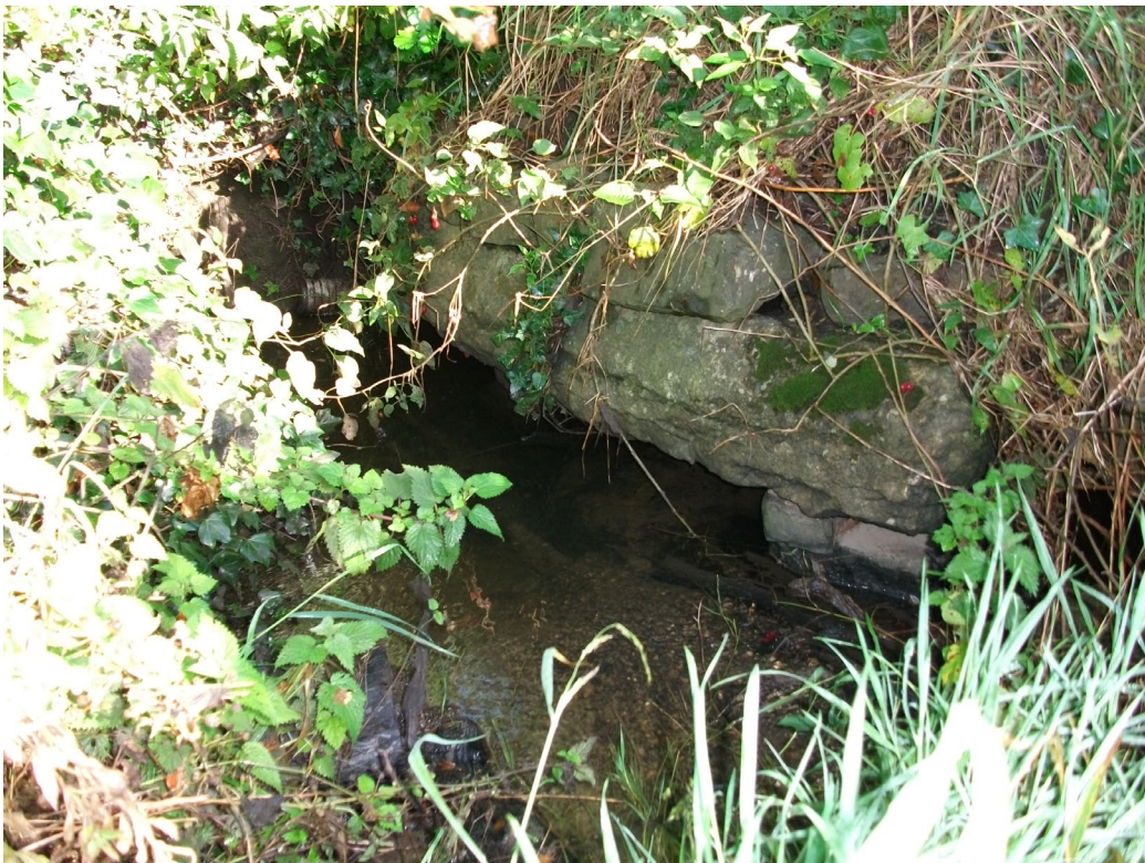
Figure 3.7: Upstream view of existing stone culvert Ch 5113
