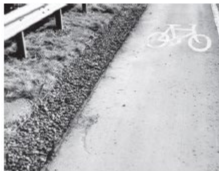
Figure 2.5: Typical Filter Drain
