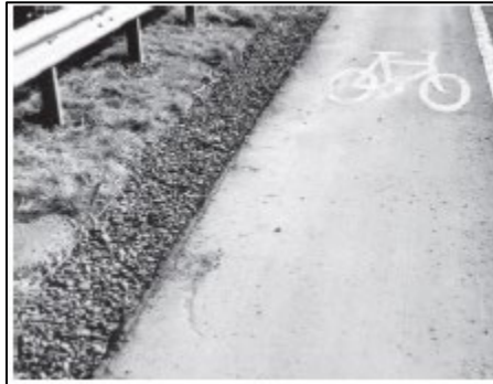
Figure 4.3: Typical Filter Drain
